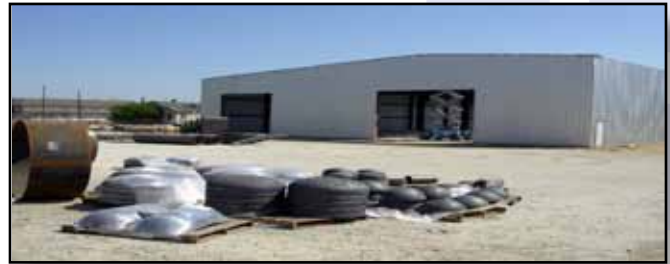
NTPV is adding 10,000 square feet to its current 20,000-square-foot facility.
